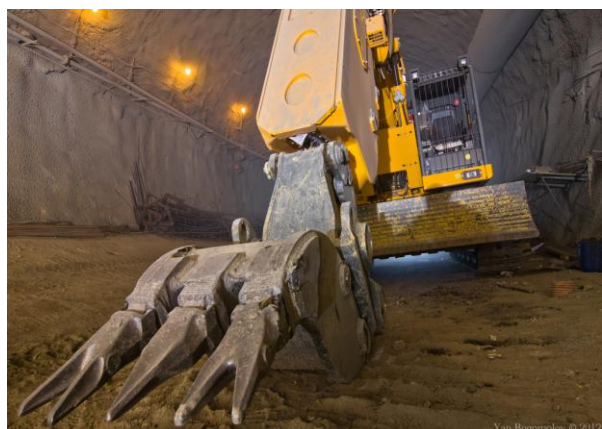
Equipment in the tunnel
